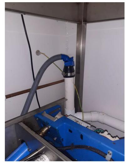
The Grey hose from the service pump is going to an upstand that has been sealed.
