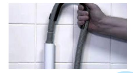
Here is an example of the grey hose being vented into the upstand, but the grey hose has been pushed below the static water level of the GreaseShield<sup>®</sup>. This will cause the water to siphon from the separation tank.
