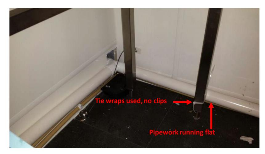
Outlet pipe **running flat** and is supported by **cable ties** to the legs of the tables.
