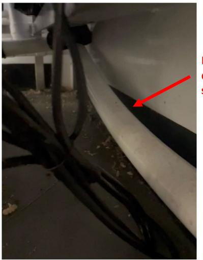
Pipe work sagging due to lack of support and clips This is what happens to pie work that is not clipped and supported properly, the pipe work begins to sag over time.
